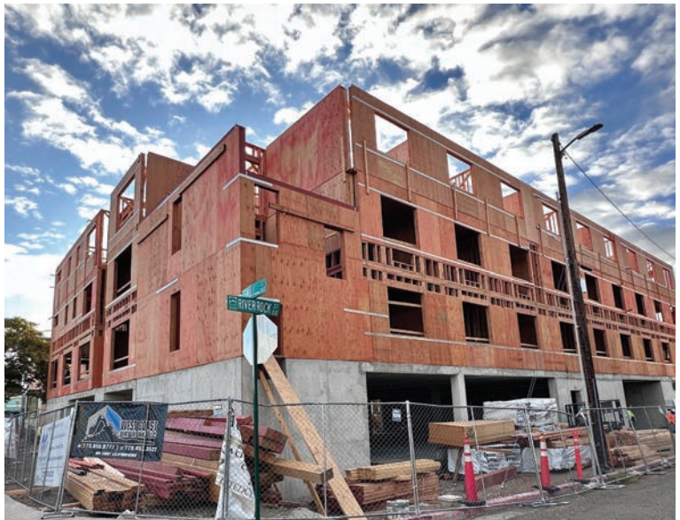
Construction at 301 State Street
